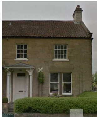
Figure 5. Example of local precedent for random coursed stone, timber windows with mock haunches and stone head and cills.
