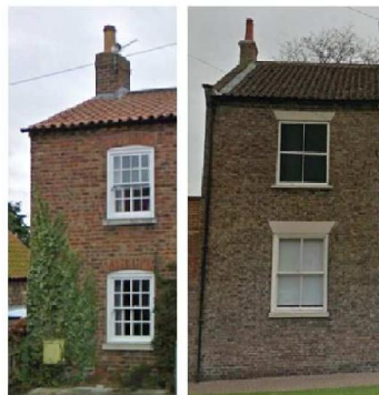
Figure 6. Example of local precedent for brickwork, Timber windows with mock haunches, shallow brick arch window head, square head, chimneys, pantiles and narrow projection eaves with spike gutters.
