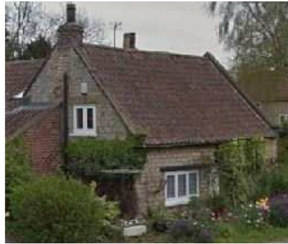
Figure 11. Local example of; - Pantile roof - Mix of stone and brickwork walls - Chimneys and gables - Small timber painted windows
