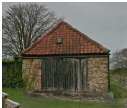
Figure 10. Example of agricultural building Typology - Pantile roof & multi brickwork
