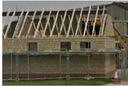
Figure 12. Local example of new reconstituted stone on brickwork plinth
