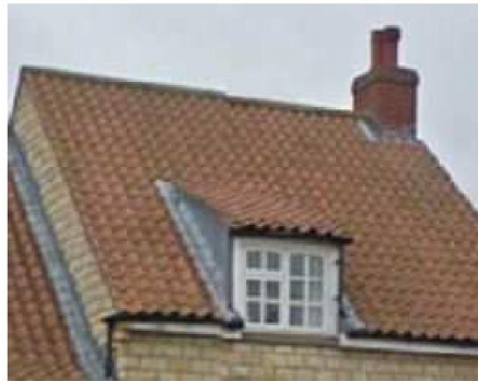
Figure 9. Local example of typical catslide dormers
